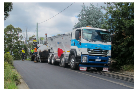
Snug falls, Road Resurfacing.
